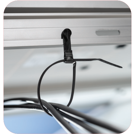
The nylon cable tie looped through the module hole is unlikely to last more than a year or two on a single-axis tracker application.
