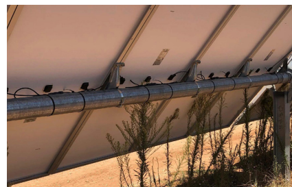
Longer ties are required for dressing wires along the torque tube. Care needs to be taken to make sure that proper materials are specified due to the high temperatures the torque tube can experience. Seen in this photo is the HellermannTyton 22 in. "Torque Tube" Solar Tie, part number 111-01196
