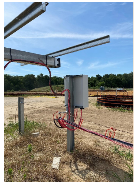
Application shows a home run properly "arrested" with T250 Solar Ties at the end of row, with drip loop and proper attachment to the post. The only additional protection recommended is UV stabilized convoluted tubing, Part: 904-00357.
