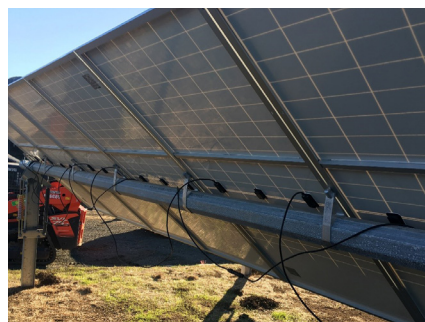
As you can see in the image, the module leads are significantly longer than needed for this application. Careful routing of the excess wires is paramount in this situation due to the lack of attachment points.
